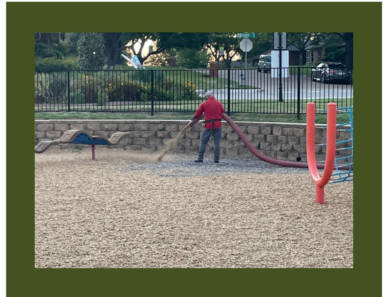
FIBAR INSTALLATION AT ALL PLAYGROUNDS
